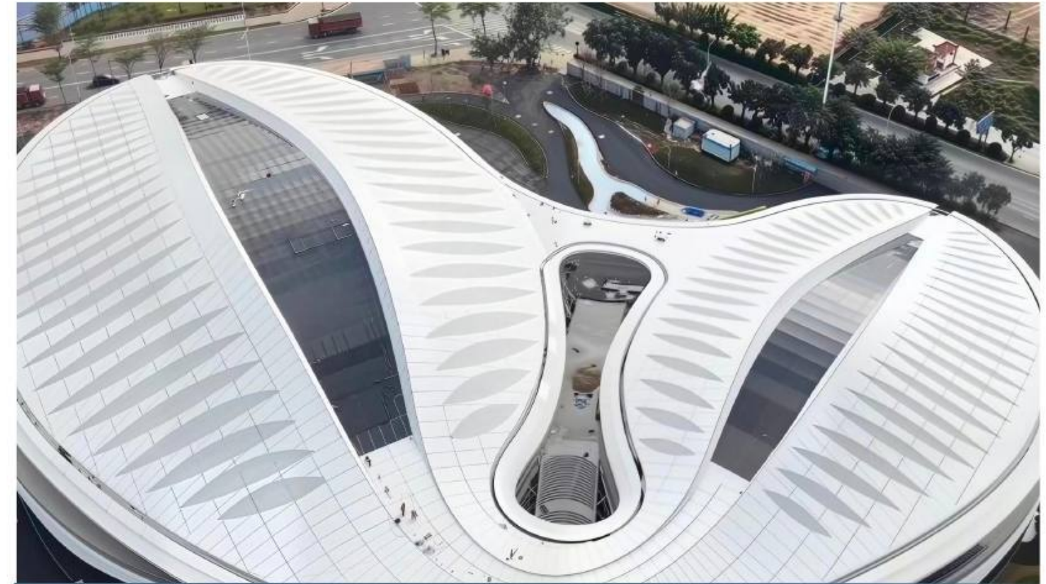
Qionghai Cultural and Sports Center (Phase II)
