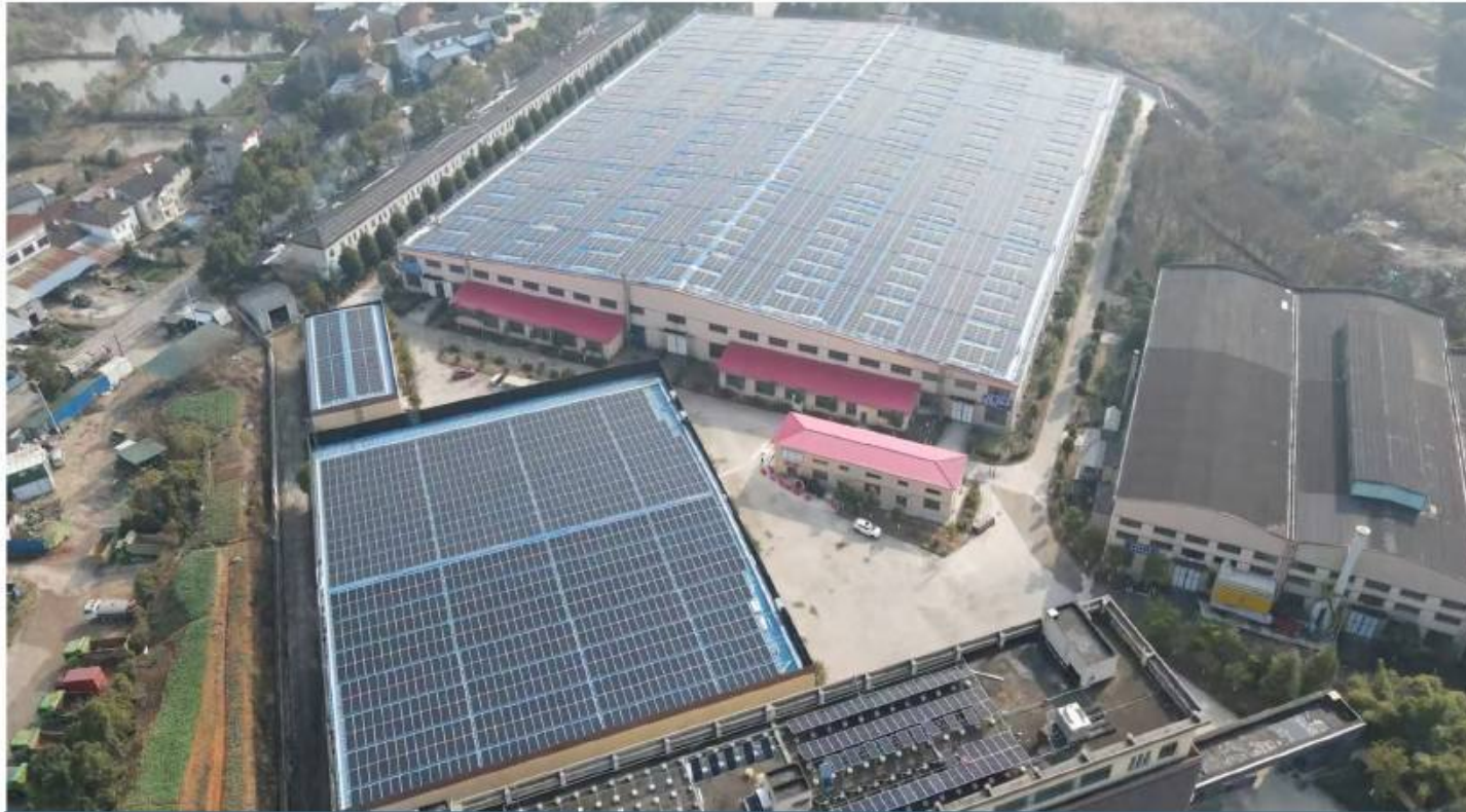
Three-Gorges Pump Industry BIPV Project (Rooftop)
